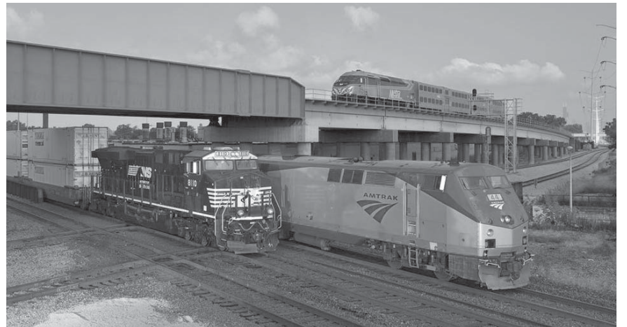
The Englewood Flyover relieves train congestion on Chicago’s south side. (Photo courtesy Norfolk Southern)
