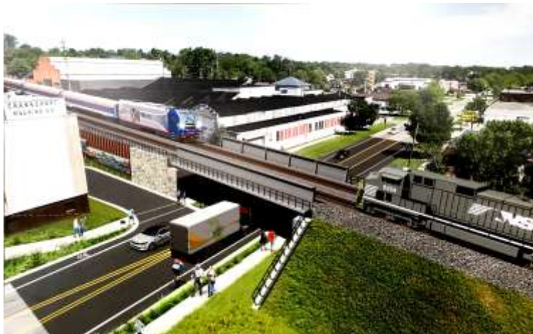
Proposed new bridge over Jackson Street. The tracks will be raised 3.5 feet to increase the clearance for road vehicles.
