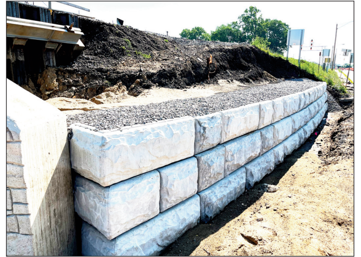
Attractive cast concrete blocks have been used for landscaping details at the bridges, both of which are located in downtown Jackson.
