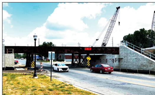
Jackson Street Bridge in June with the new abutments.
