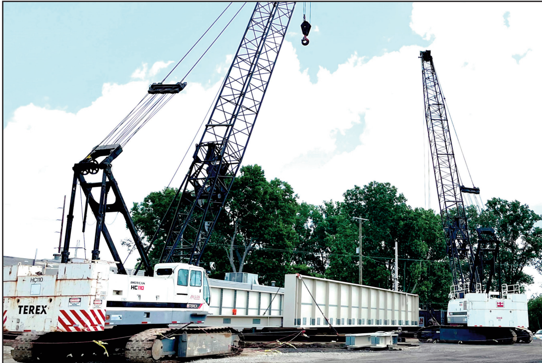
Jackson Street Bridge structure ready to be lifted into place.
