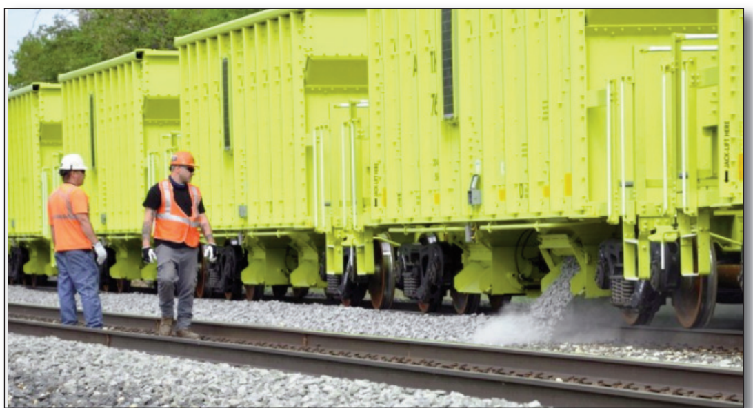
Amtrak ballast train applies additional ballast as part of track maintenance west of Jackson on May 19, 2021. (Roy Davey photo)
