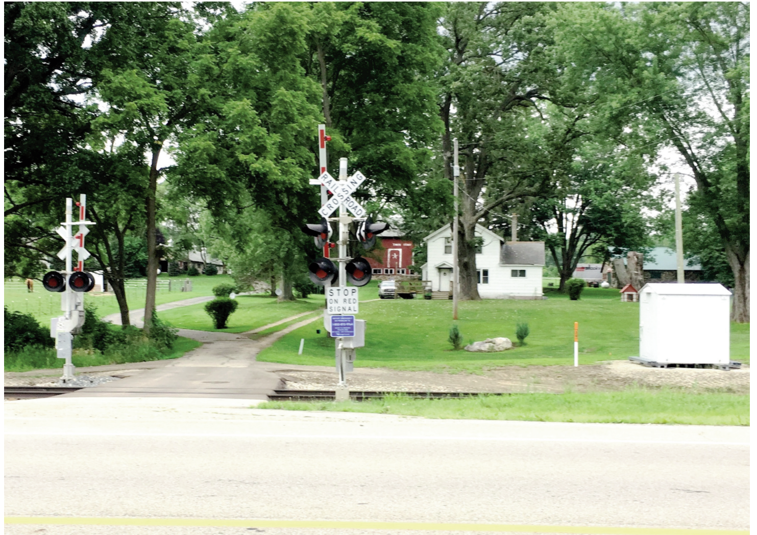
A private grade crossing to a single residence. This crossing on the Amtrak Michigan Corridor near Parma is protected by lights, bells, and crossing gates.
