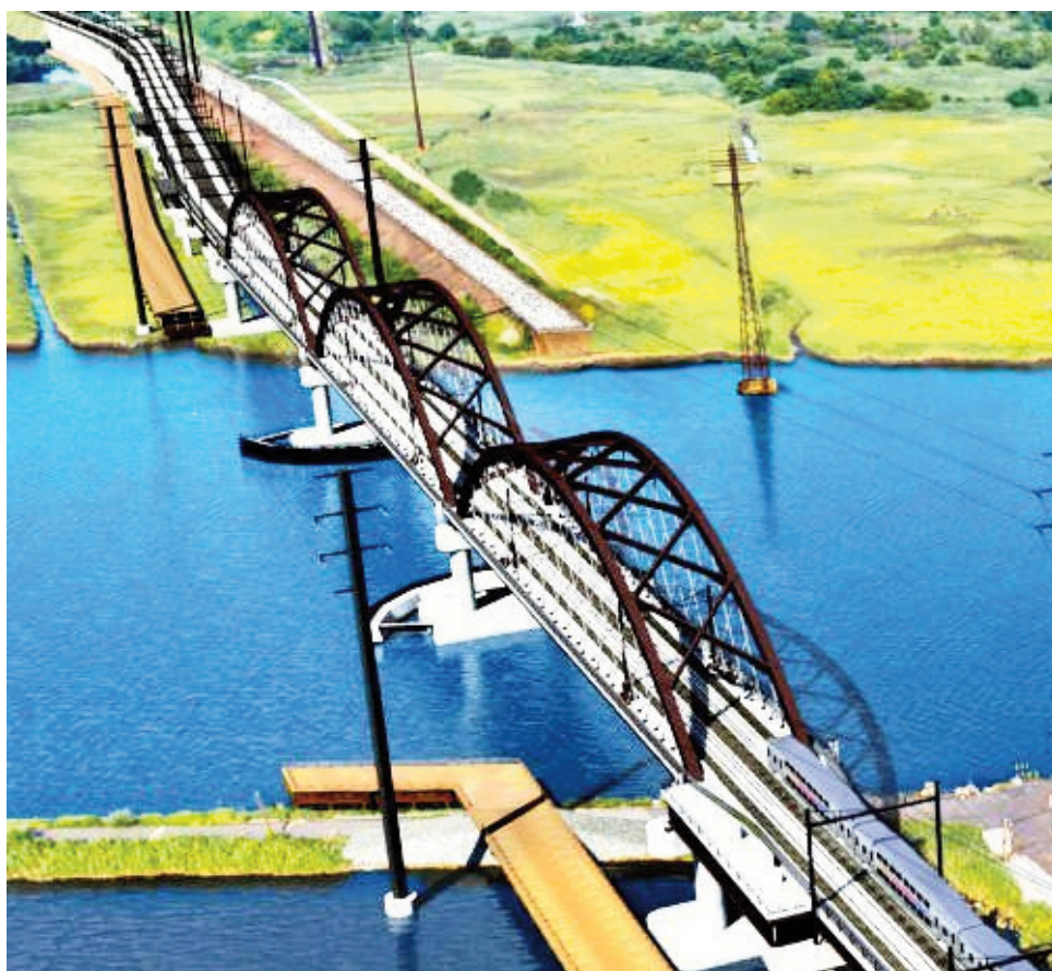
Sketch showing the proposed new Portal Bridge over the Hackensack River west of the Secaucus station in New Jersey on the Northeast Corridor. The new three-span bridge will be built alongside the 112-year-old, 961-foot, turn bridge originally built by the Pennsylvania Railroad and opened in 1910. The new bridge will be fixed in place and provide enough clearance over the river without having to open for river traffic. The old bridge will be removed after the new bridge is in service. (Amtrak sketch)
