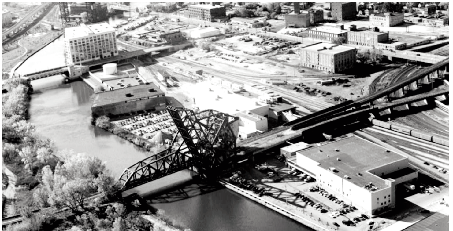
The double-track St. Charles Air Line (SCAL) Chicago River Bridge (the bridge in the closed position) and the elevated SCAL are shown in this aerial photo about 1960. This view is looking to the southwest with the south part of what is now Amtrak's Chicago rail yard in the center of the photo and the Dan Ryan Expressway (I-90/94) in the background. According to Wikipedia, the bridge is a Strauss Trunnion bascule bridge, originally 260 feet long when built in 1919, the longest such design in the world at that time. When the Chicago River was channelized in 1930, the bridge was shortened to 220 feet in length. The St. Charles Air Line is about 2 miles in length and was built by several railroad companies as an east-west connector to cross over several north-south railroads and the Chicago River. (Library of Congress photo)
