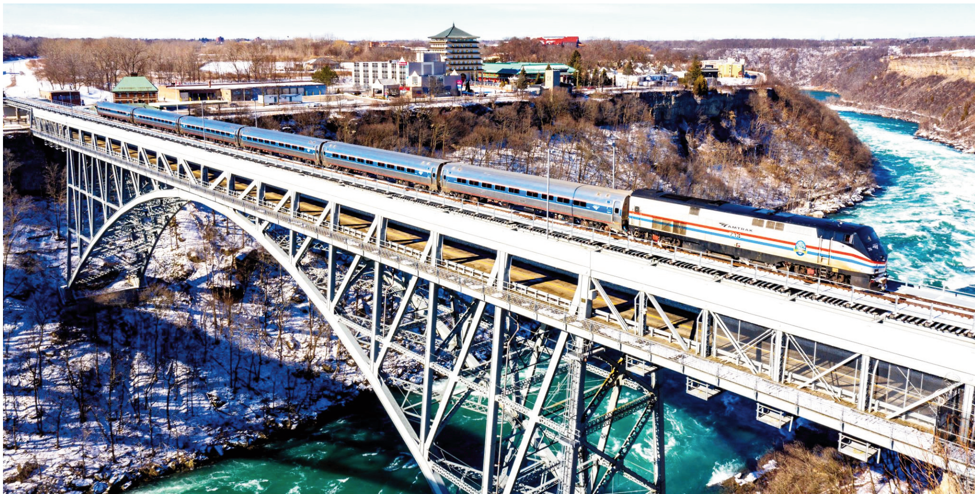
The Maple Leaf crosses on the CN Whirlpool Rapids bridge over the Niagara River Gorge. The Via Rail Station for Niagara Falls, Ontario and the Amtrak Station for Niagara Falls New York are at near each end of the bridge, about 1,500 feet apart. The parallel, unused Michigan Central bridge is about 250 feet upriver, just to the left outside of the photo. (Amtrak photo)
