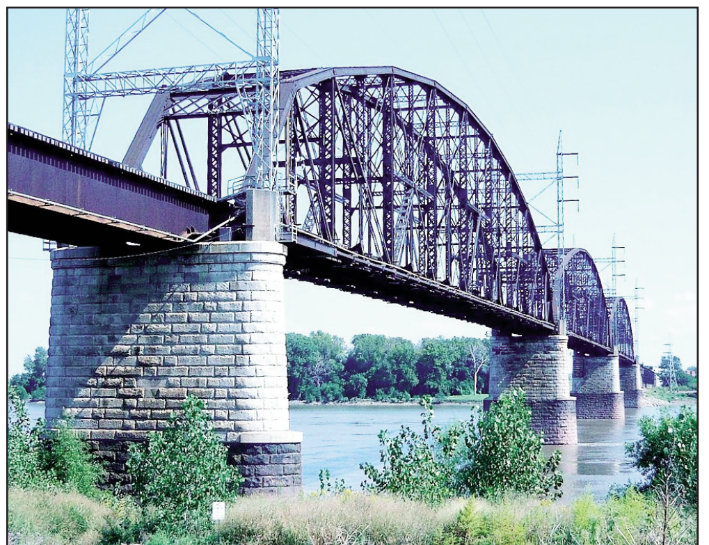
The massive Merchant Bridge at St Louis was opened in May of 1889. It carries dozens of freight and Amtrak trains each day over the Mississippi River and is being rebuilt with new spans to remove load, speed, and clearance restrictions. (Wikipedia Commons)
