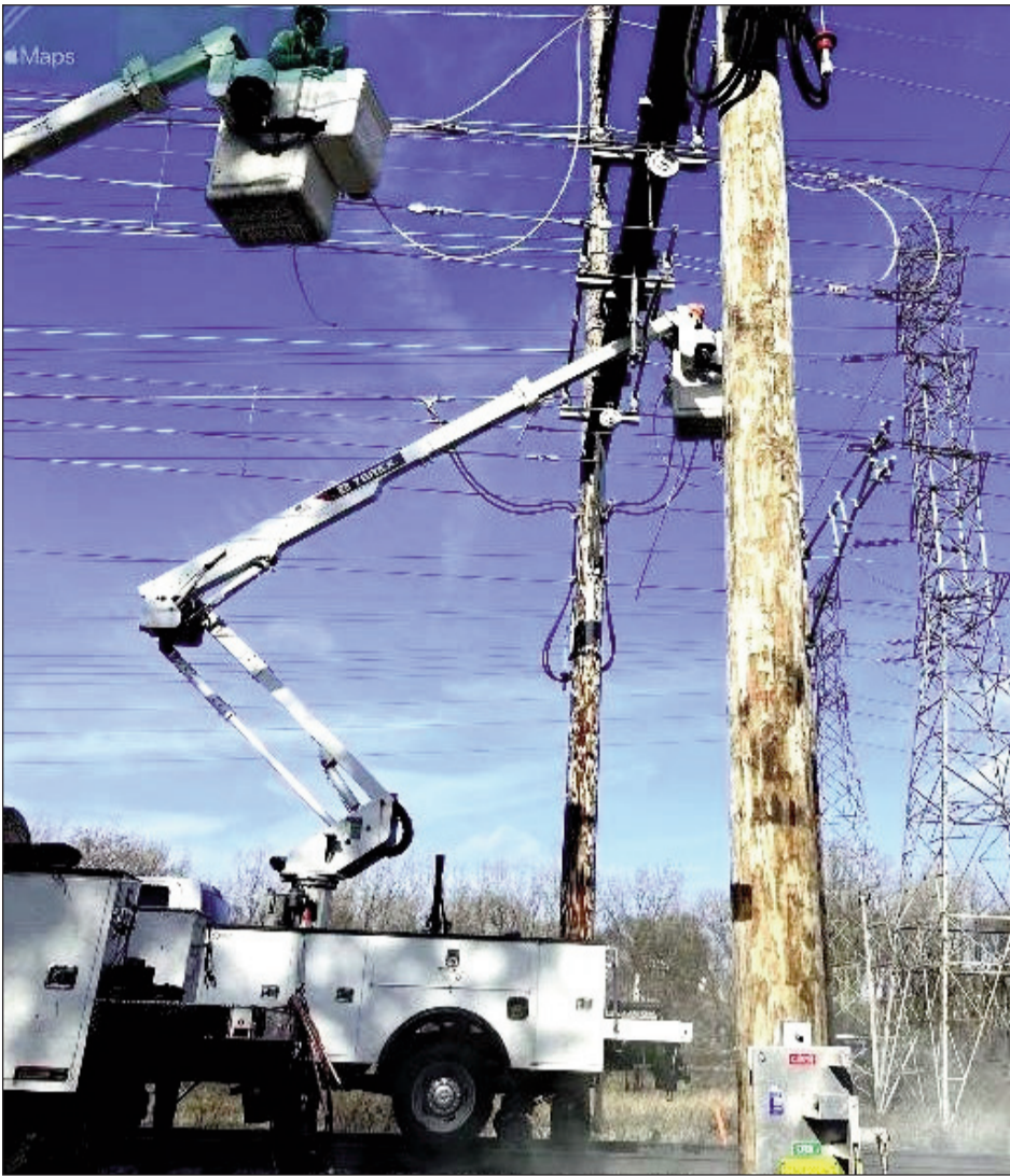
Catenary upgrade on the South Shore railroad. (South Shore photo)
