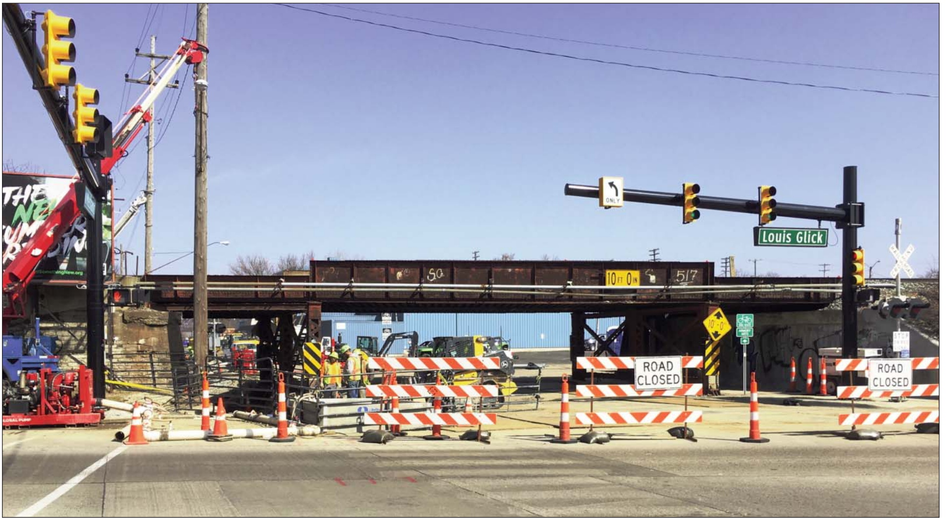
Looking north at the Mechanic Street Bridge on March 17, 2021.
