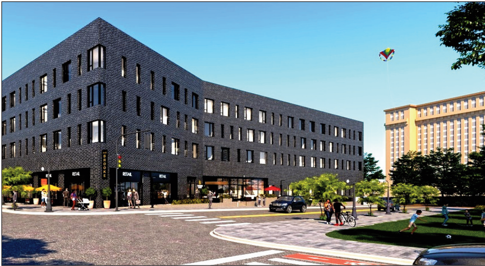
Above, the newly opened Brooke on Bradley, a $23 million apartment house investment on the corner of Bagley Street and 16th Street, is a result of the Michigan Central redevelopment. These apartments are within walking distance of MCS and the NewLab. MCS can be seen in the right rear of the photo. (Brooke on Bradley photo.)
