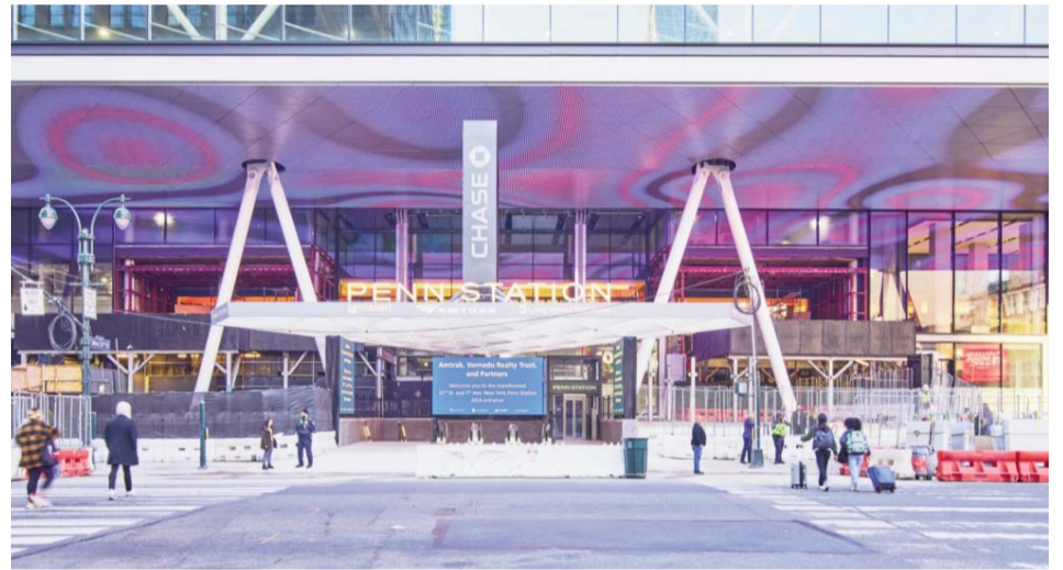
The Seventh Avenue entrance down into Penn Station, a subterranean den of crowded corridors, shops, and fast food eateries that is seemingly always disrupted by endless construction work. It all lies under the 2 Penn Plaza office tower and Madison Square Garden. (Fernando Sandoval/MW photo, via Amtrak)
