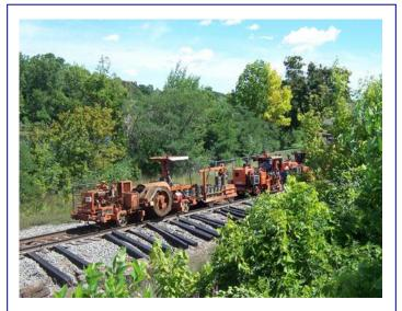
This was the scene last month as Norfolk Southern track crews of 75 men or more worked on the 135 mile segment between Ypsilanti and Kalamazoo replacing ties, smoothing the track, and improving grade crossings. The repairs have resulted in the lifting of speed restrictions that were slowing Wolverine trains between Ypsilanti and Battle Creek.
